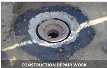
CONSTRUCTION REPAIR WORK
