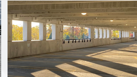
HUDSON STREET PARKING GARAGE
