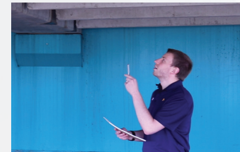
PARKING GARAGE CONDITION APPRAISAL
