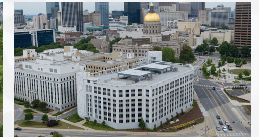
GEORGIA STATE CAPITOL PARKING GARAGE
