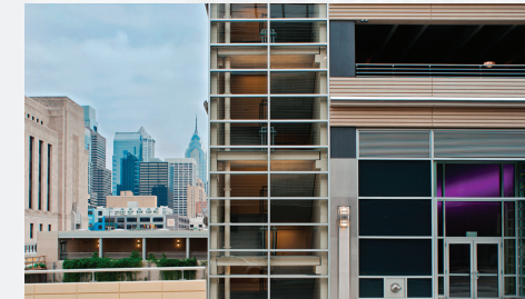
CIRA SOUTH PARKING GARAGE
