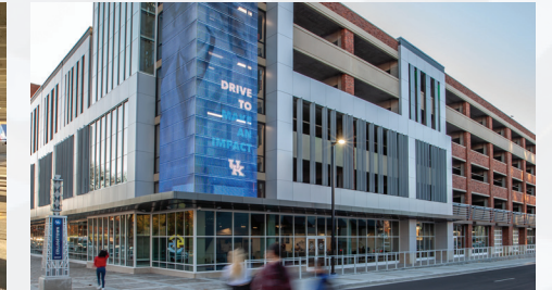
UNIVERSITY OF KENTUCKY PARKING GARAGE
