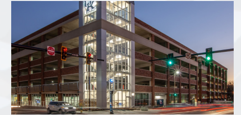
UNIVERSITY OF KENTUCKY PARKING GARAGE
