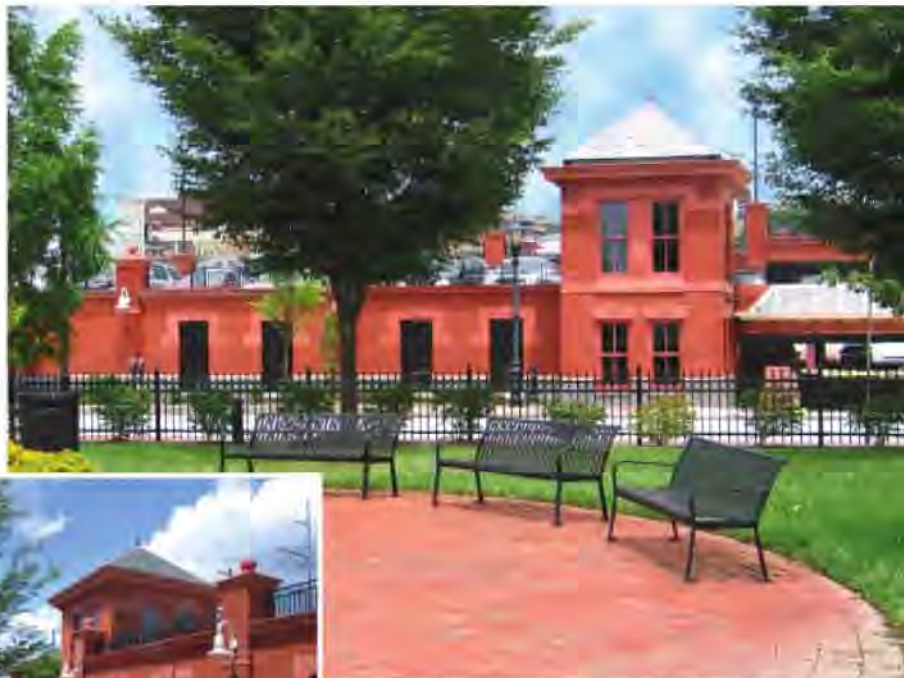
The Riverfront parking garage in Wilmington, Del., serves Amtrak riders, visitors and employees of a nearby corporate headquarters building. On weekends, visitors use the garage for special events at Riverfront Plaza, located directly across the street from the garage.
