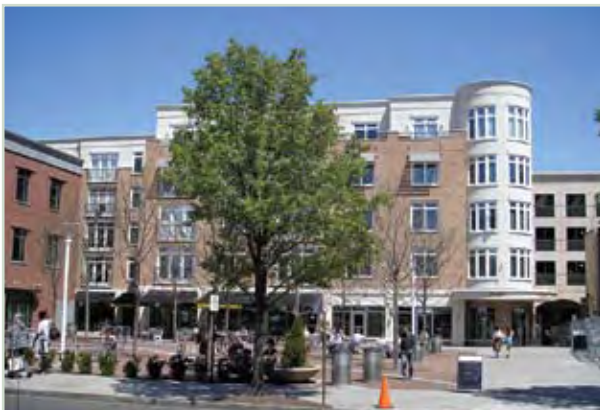
Downtown – Princeton The Princeton Downtown Redevelopment Project includes a 500-space parking facility which features housing at the front and retail space at the ground level.
