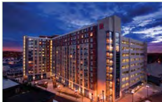
Education – Morris Street The Morris Street Parking Garage in New Brunswick, N.J., serves the adjacent student housing in Rockoff Hall at Rutgers University.
