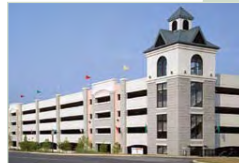
Healthcare – duPont The Alfred I. duPont Hospital for Children parking structure was designed to resemble a castle, and features a courtyard to provide an inviting space for patients, visitors and employees.
